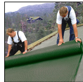
Figure 21. Rolling out Membrane Source: Safeguard
