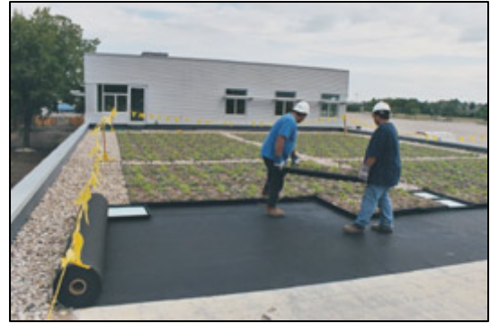
Figure 28. Workers Placing Filter Fleece in Preparation for Soil Layer Source: G-Sky
